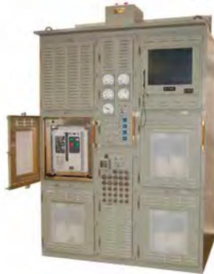
Leonardo DRS is a leader in providing Low Voltage Switchboards and load centers to military or marine grade specifications. Utilized on the latest U.S. Navy ships for power distribution, the military hardened switchgear is designed to withstand rugged maritime conditions for the life of the ship.
